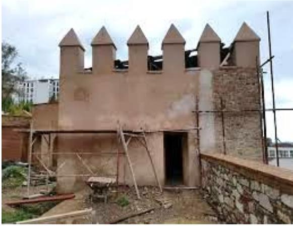
Fig. 08. Restoration work (plastering) on part of the Bastion.
