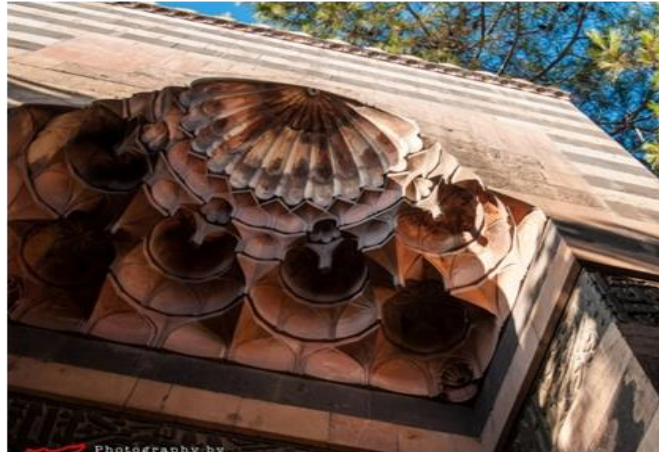
Figure 12. View of the dome of the main entrance of the Madrasa Al Jaqmaqya in Damascus.
